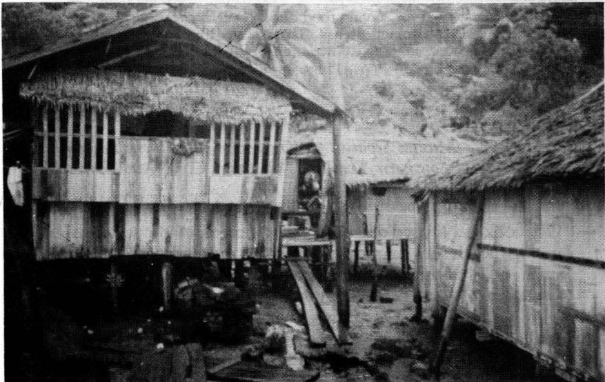
A typical Yakan house in Gaunan, Maluso made of wood, nipa , and bamboo. The main house is separated from the kitchen. [Photo by Ermina K. Mariano]
