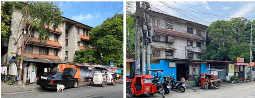
Figure 37: Sikatuna BLISS - informal additions
