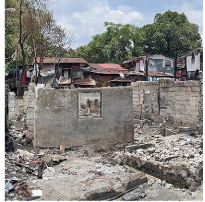
Aftermath of the fire
