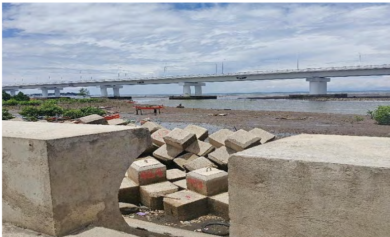
Figure 10. The current shoreline in Barangay Talomo, with the dike and boulders, and the depleted mangrove forest
